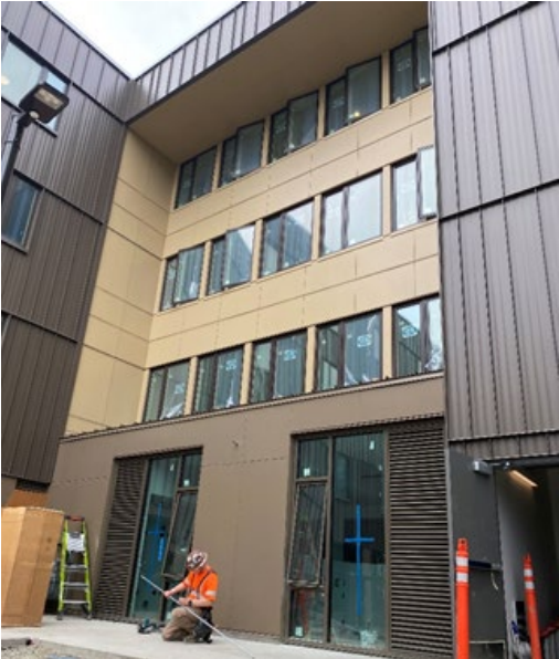
South wall of west courtyard
