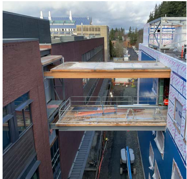
Figure 2: Bridge to CF
