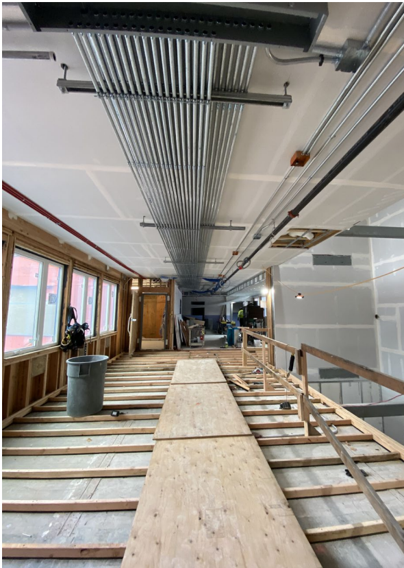
Second floor in elevator lobby, middle of the building, March 8, 2021
