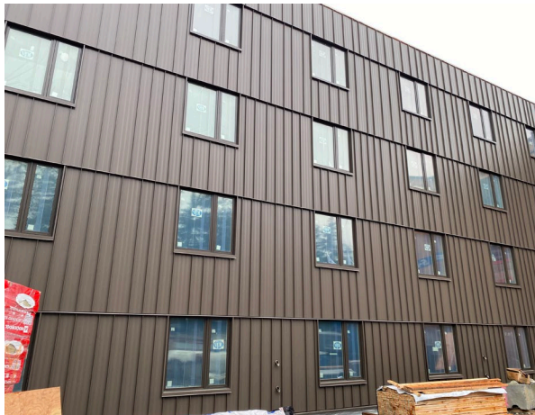
New siding and windows being installed, March 8, 2021
