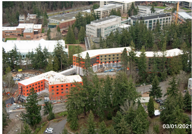
Aerial photograph by Dan Bigelow, SkyShots Aerial Photography, March 1, 2021
