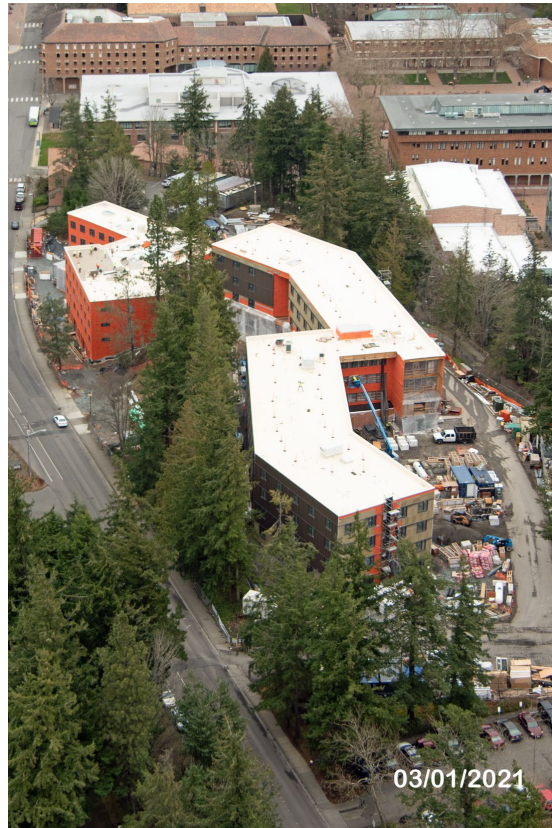
Aerial photograph by Dan Bigelow, SkyShots Aerial Photography, March 1, 2021
