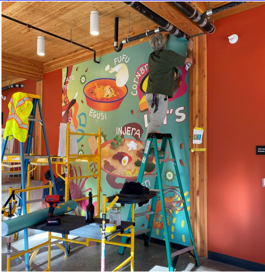
Graphics being installed on the fourth floor
