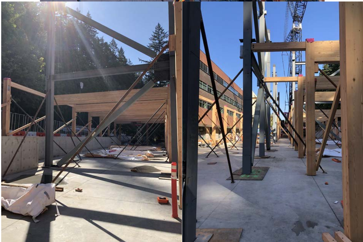
Construction of mass timber and steel structure
