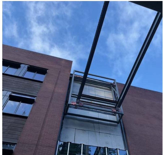
Figure 2: Steel installed for bridge to CF
