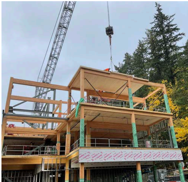
Figure 1: CLT installation on upper floors
