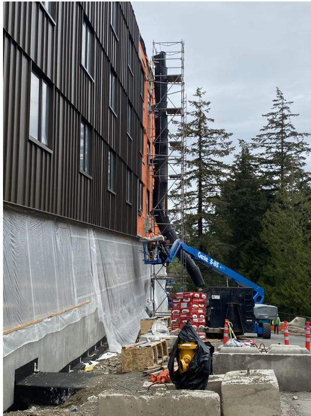
Exterior siding installation, May 5, 2021
