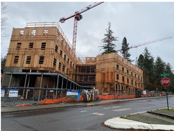
View of north portion from street, 12/15/20
