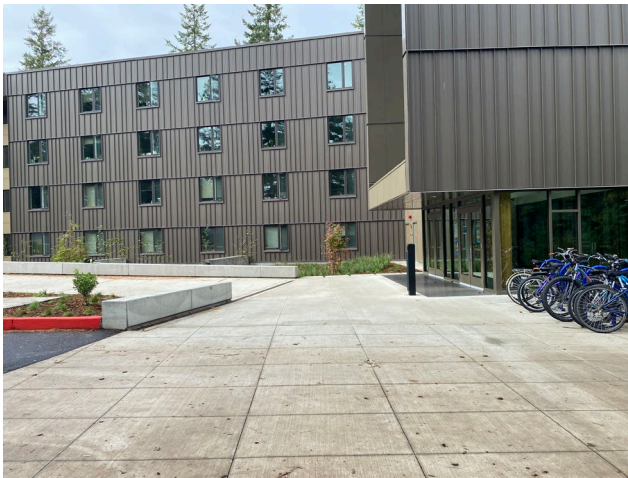
Entrance at south end of building
