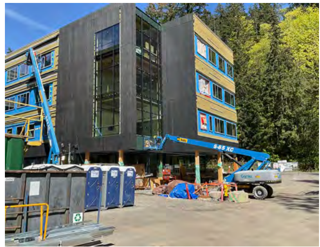
Figure 2: Southwest corner of building siding installation
