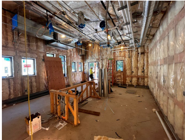
Figure 8: Construction progress in Teaching Kitchen
