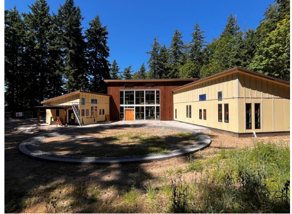
Figure 7: Exterior siding and windows
