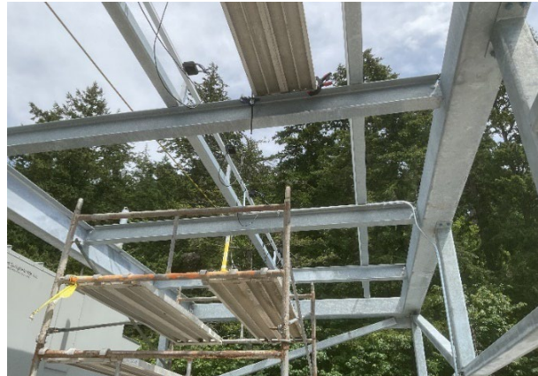
Figure 2: Solar panel supports on roof
