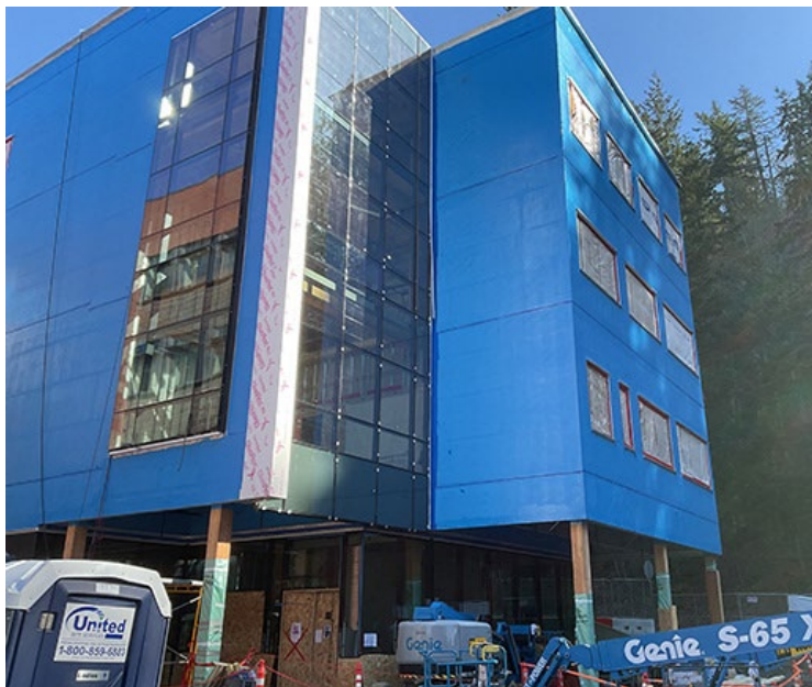
Figure 1: Southwest corner of the building
